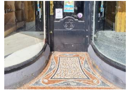
Figure 12 A curved lobby with mosaic tiling.
