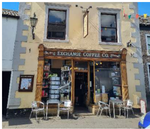
Figure 4 A restored traditional shopfront with carved timber details and hanging sign.
