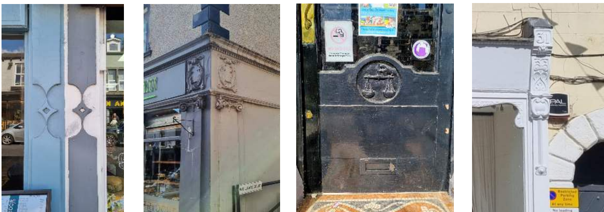
Figure 8 Decorative features retained on shops in Clitheroe.
