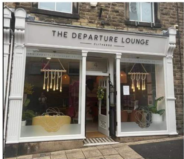
Figure 7 The same shop today showing some replaced materials and loss of the cornice, but the same basic design preserving character.
