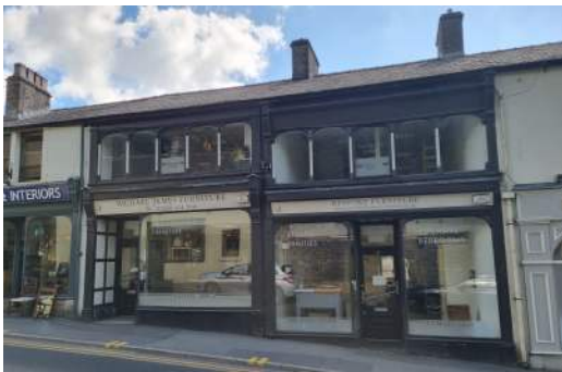
Figure 2 Unusual first-floor arcaded shop windows.
