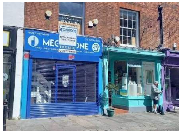
Figure 15 A traditional shopfront concealed by a modern roller shutter and insensitive signage.
