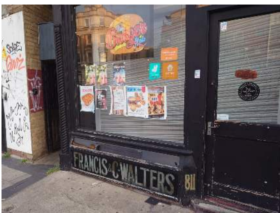
Figure 14 A grade II listed shop with internal shuttering that does not obscure original features.
