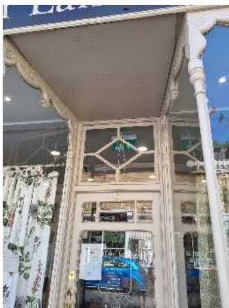
Figure 3 Cast iron decorative details.
