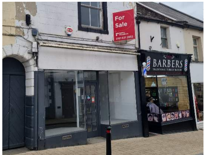
Figure 11 Divided windows have been lost and replaced by plain sheets of glass
