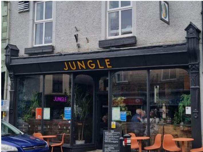
Figure 8 A modest timber fascia contained by corbels, with tasteful signage applied as single letters.
